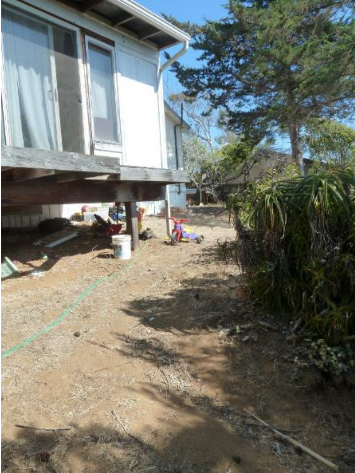
Figure 4. Runoff from Lomaland property roof drains and impervious hard surfaces run into Drainage Basins G, I, and the Upper Parking Lot in Basin J. This runoff should be directed to Lomaland Drive.
