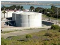
*"During World War II, the DOD installed concrete 'splinter' walls around the aboveground tanks to protect them from bomb shrapnel."*
