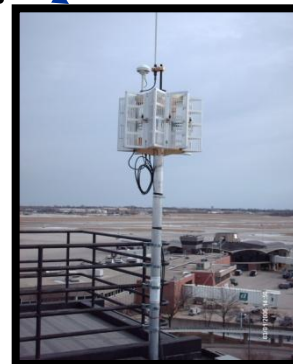
Passive Secondary Surveillance Radar (PASSUR)
